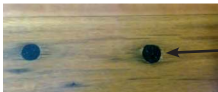
Black resin filled bolt holes
