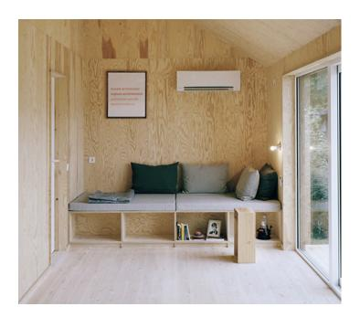
Interior plywood can have face grades of AC or BB. A grade faces are designed for clear finishing while a B grade face is designed for painting.
