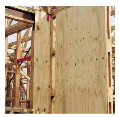
Austim can supply Structural plywood in the following stress grades F8, F11, F14 & F17, untreated or treated. H2 glue line, H3 Envelope or H3 Veneer treated Structural plywoods are available upon request.
