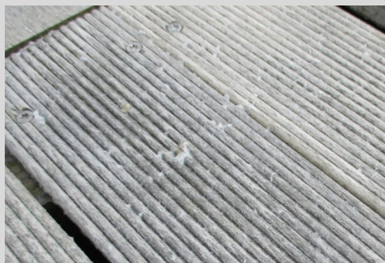
Fibres may get trapped in ribbed surface profiling.
