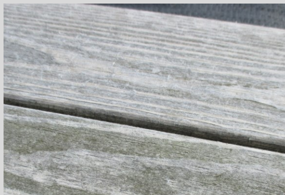
Natural occurring surface fibres on decking.
