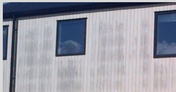
A New-Zealand housing project with a very distinct batten silhouette showing in the cladding surface.
